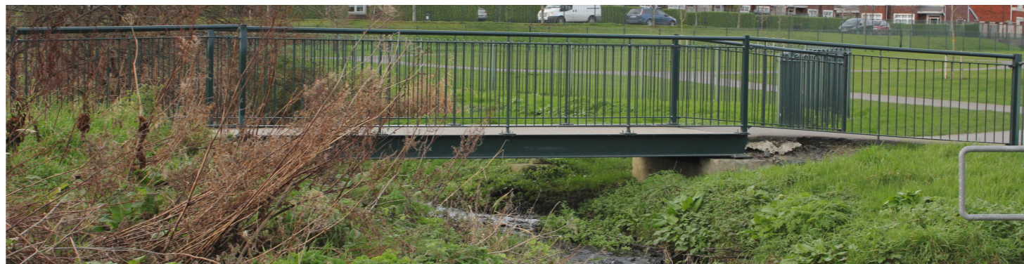
River Bridge Crossing
