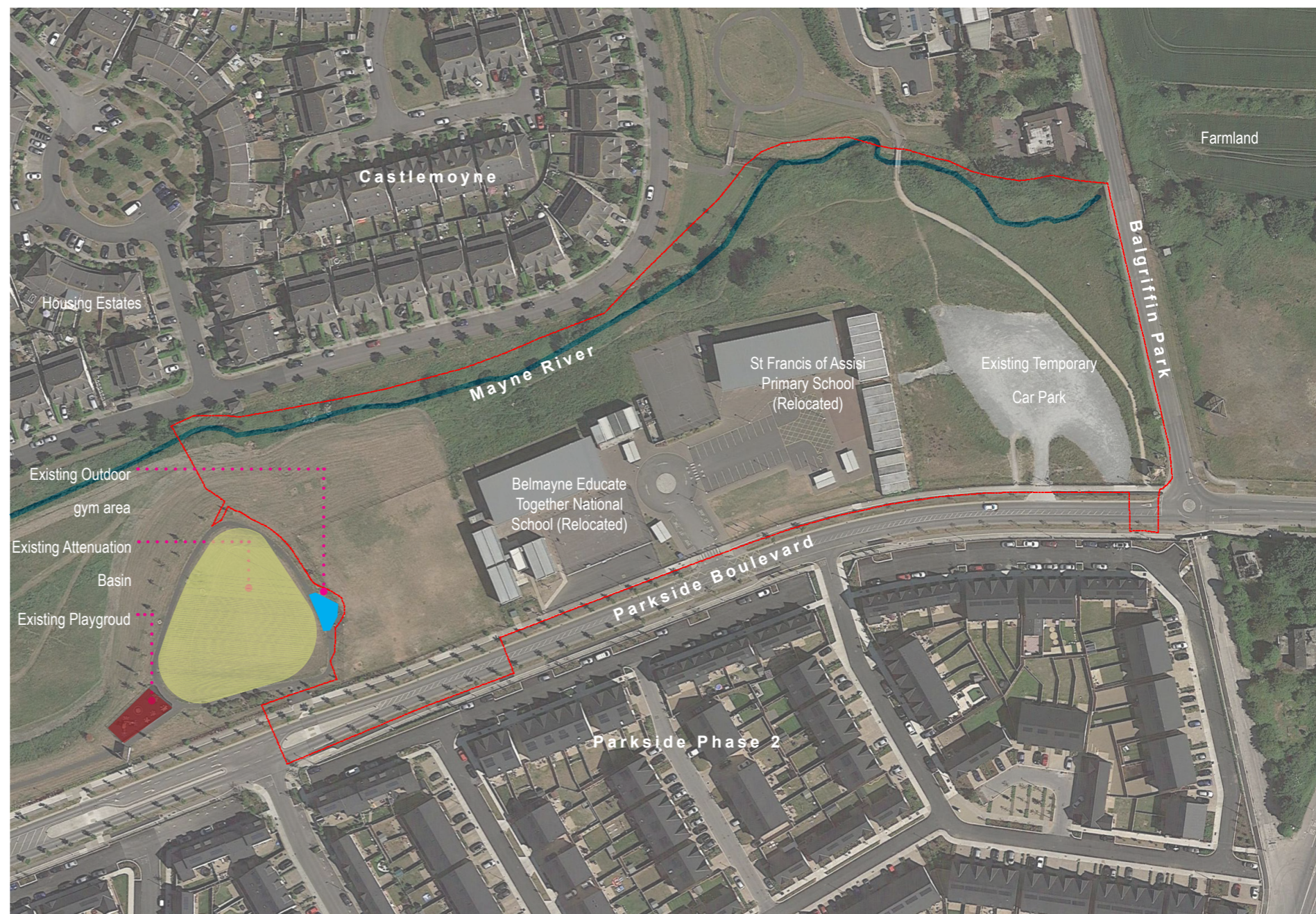
Aerial photograph of the site taken from Google Earth 2019.
