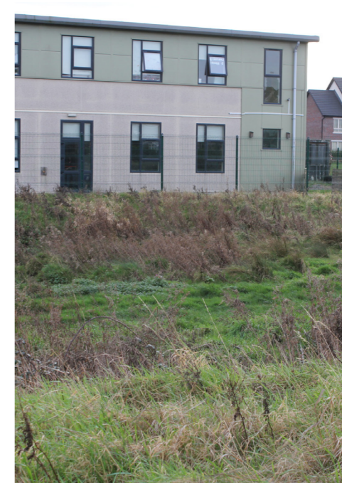
River Embankments North of School
